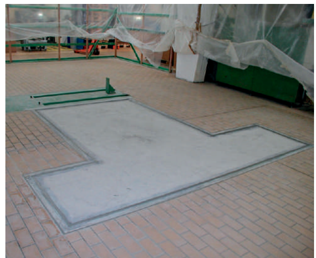
Cast foundation block
