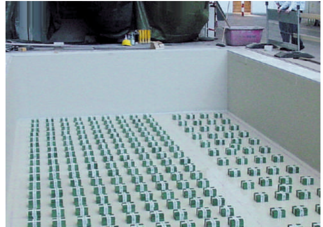
Foundation pit with Bilz insulation pads laid out
